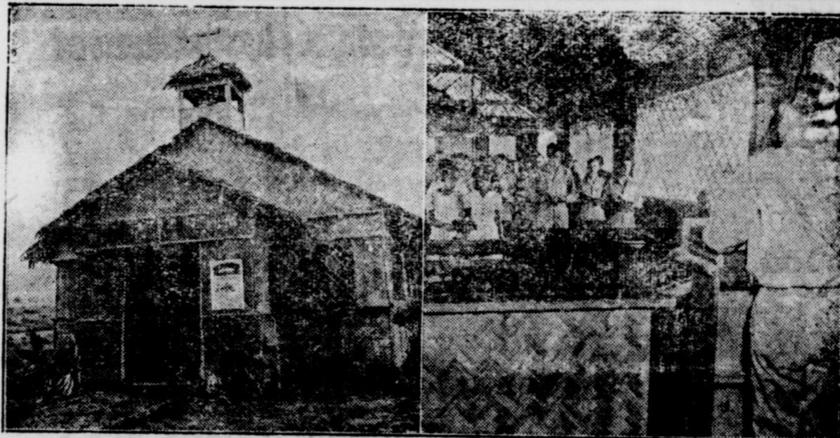
ROOSEVELT MEMORIAL CHAPEL IN THE PHILIPPINES—This quaint bamboo house of worship in Grace Park, Manila, was built by soldiers of the 513th AAA Gun Battalion and dedicated to the memory of President Roosevelt. Right, Army Chaplain Paul M. Bourne conducting the dedication services. The chapel will be given to the native Filipinos upon the withdrawal of American troops.
