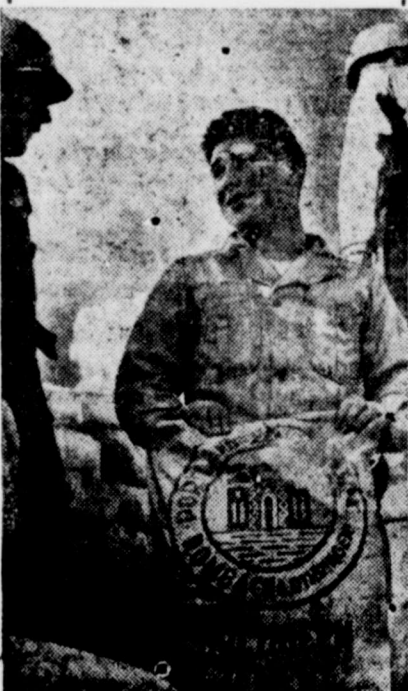
Signal Corps Photo Pvt. Isidore Sack, New York, displays German cement captured in France and being used to build road to an American airport. Confiscated materials help the U. S. war effort but War Bonds pay for the vast quantity of material necessary for victory. U. S. Treasury Department
