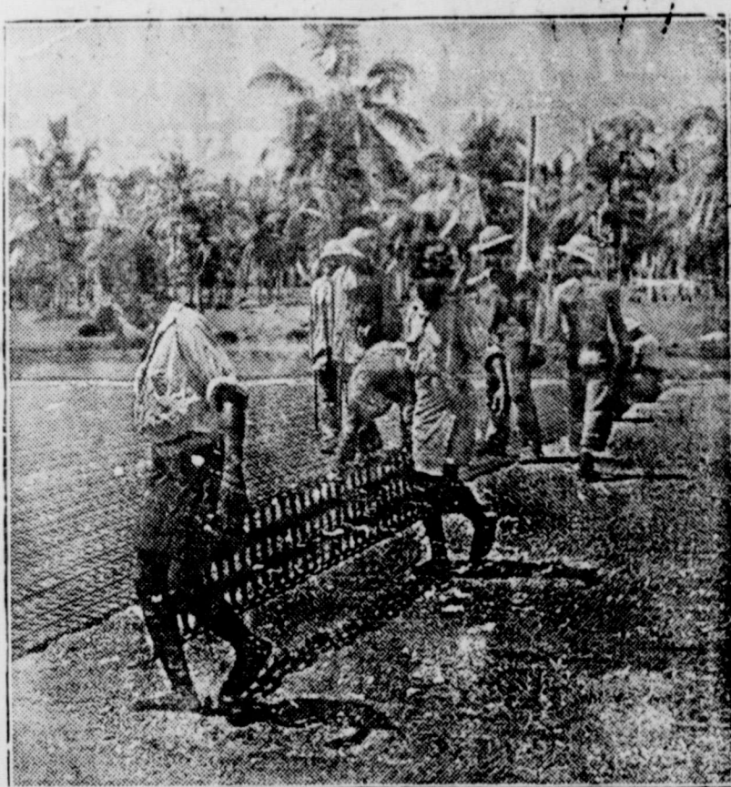
Bureau of Public Relations, U. S. War Department JUNGLE AIR FIELD IN SOUTHWEST PACIFIC—Utilizing native materials and labor, U. S. Aviation Engineers have carved a mile-long runway out of the heart of the jungle. Natives are shown laying the portable steel landing mat under the direction of the Engineers. The foundation is a bed of crushed coral which is locally available in plentiful quantities.
