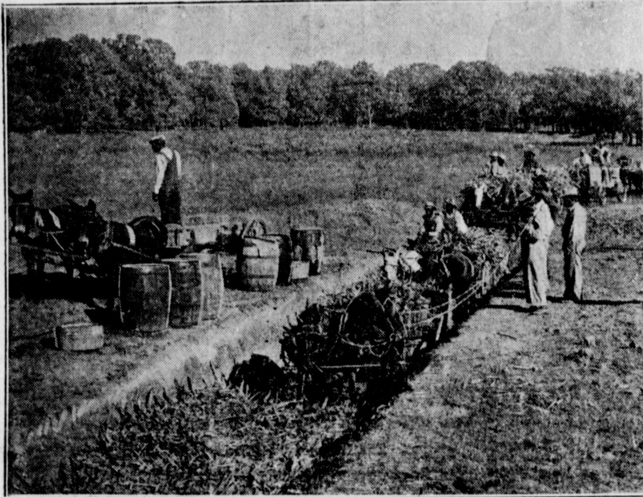
TRENCH SILO BUILDING PROGRAM TO HELP FARMERS
