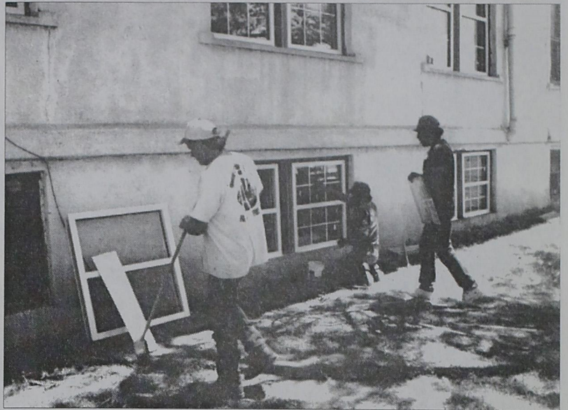
WORKERS RESTORING THE OUTSIDE OF THE CHURCH BUILDING
