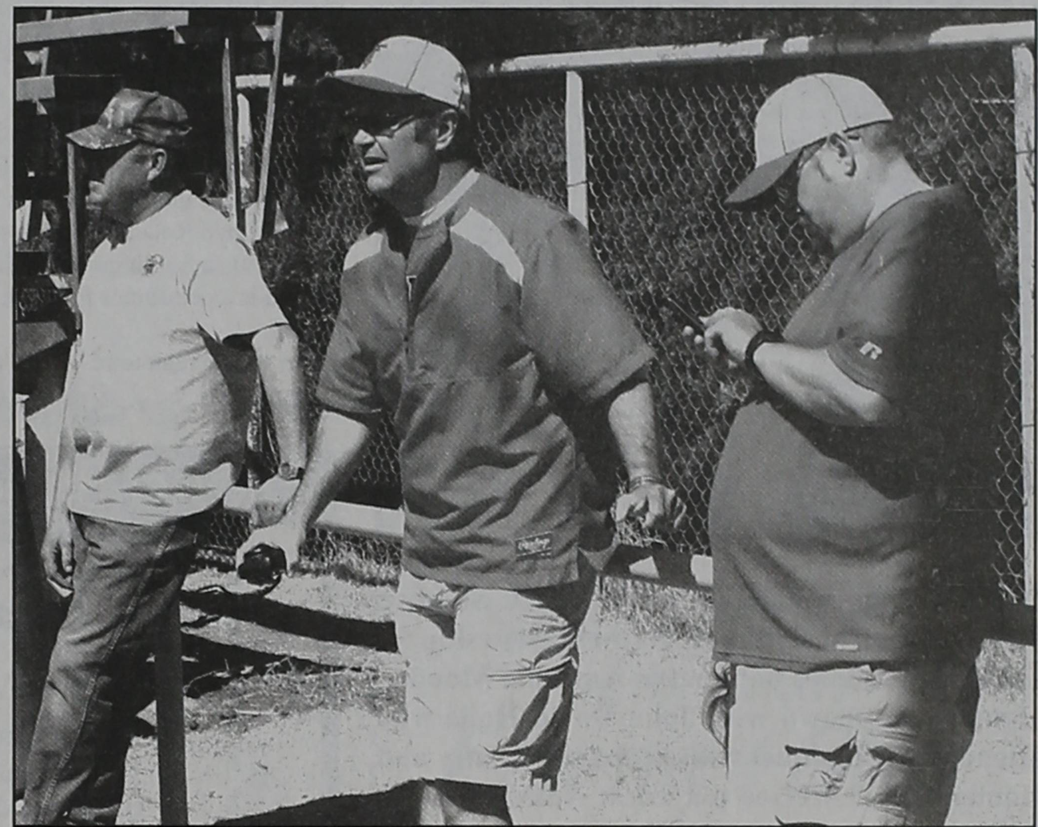
ron carr photo Chuck Teague, l-r, Mark Sundre, and Chris Morrow try out the new "leaning rail" that Chuck installed at the baseball field for restless dads to lean against during Chieftain games. Some dads just do not like to sit still in the stands.
