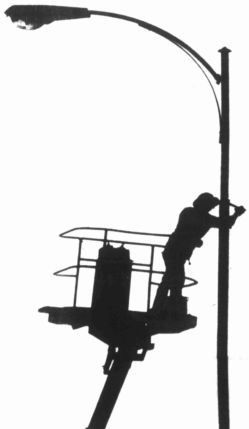
NEARING THE END — Light standard painter Richard Constantino, who works for an Abilene firm, stretches to paint a light standard in downtown San Angelo early Monday morning. His crew is nearing the end of their project to paint all the light standards in the San Angelo area — over 1,300 — with only about 100 to go.
