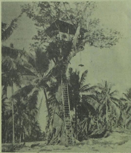
CONTROL TOWER...This was a MAG II Operation Control Tower on Espiritu Santo in the Pacific during WWII. It was built in a mahogany tree. The GIs used whatever was available in the area.
