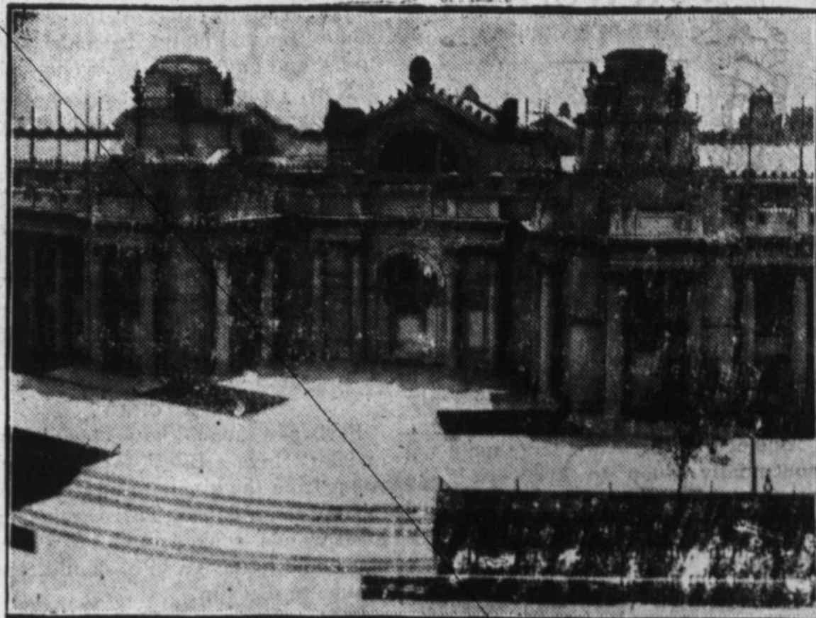
SUNKEN ENTRANCE PALACE OF ELECTRICITY, WORLD'S FAIR, ST. LOUIS.
