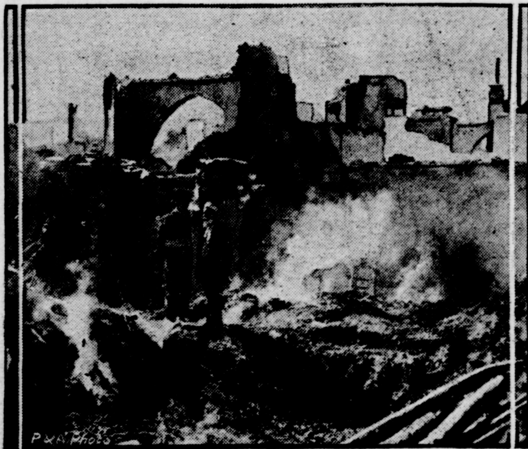
The shelling of the beautiful city of Damascus by the French troops under command of General Sarrail shocked the entire world and resulted in the recall of the general. Two thousand persons are said to have been killed. This photograph shows the totally ruined appearance of the city after the shelling.
