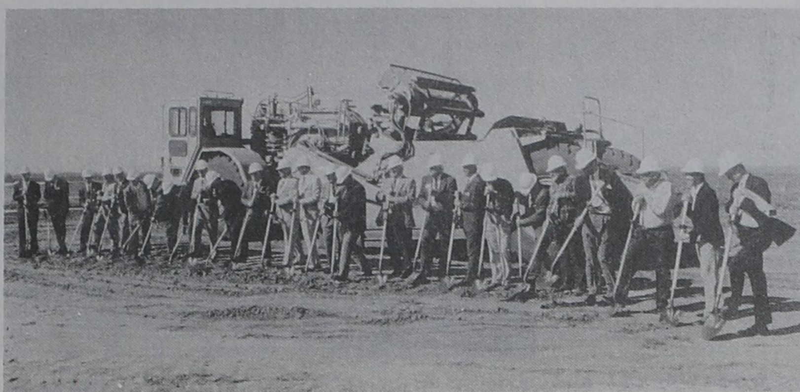
NEW POWER PLANT... Ground is broken for the $145 million Mustang Station being constructed near Denver City, by the board of directors of Golden Spread Electric Cooperative, representatives of bankers CoBank and Societe Generale, and by Yoakum County Judge Dallas Brewer and Stan David, city manager of Denver City.
