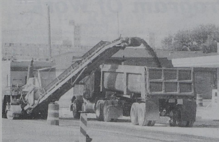
CHEWING UP PAVEMENT....TX/DOT contractors are shown here chewing up the asphalt on the west side of Main Street the first week in August 1997 in preparation for repaving, a part of the Main Street renovation project.
