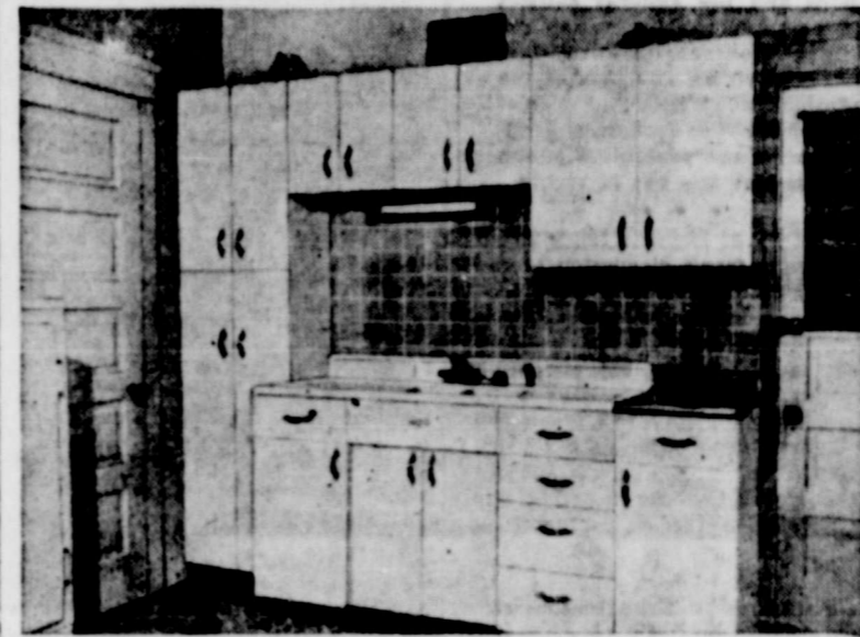
No need to pity the homemaker now. Her modern kitchen saves many hours of hard work. The cost was low because installation of standard steel cabinets and cabinet sink was done quickly without expensive room alterations. Not even the plumbing was changed. Wall tile and a light above the sink are helpful features. There is a lot of work surface on the porcelain enameled top of the steel cabinet sink and on the adjoining base cabinet top. There's lots of storage space inside, too. Dishes are washed in the sink bowl and the dishpan has been consigned to the trash pile.
