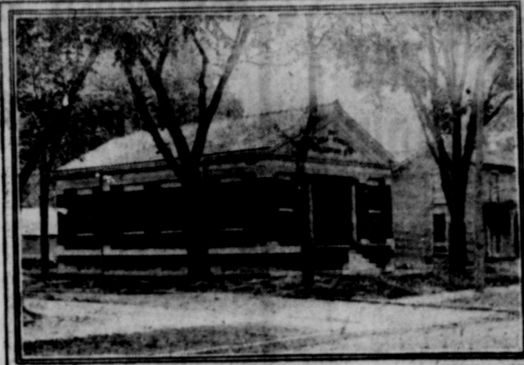
BRYAN-BENNETT LIBRARY BUILDING AT SALEM, ILL.
