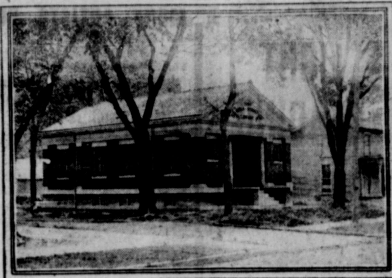
BRYAN-BENNETT LIBRARY BUILDING AT SALEM, ILL.
