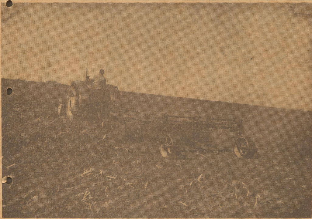
LAND LEVELLING is done with many types of equipment, all the way from a hand-made wooden "float" to a large blade-type machine like this which has both a planing and dirt moving action. This is a scene in Oklahoma Lane.
