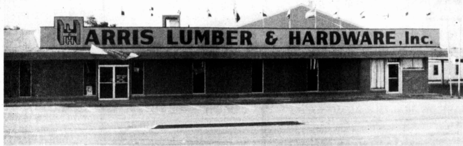
ONE-STOP SHOPPING — Harris Lumber and Hardware, 1609 E. 4th, has just completed the remodeling of its store, and installed a new warehouse to better serve the needs of Big Spring's homeowners. (Photo By Danny Valdes)
