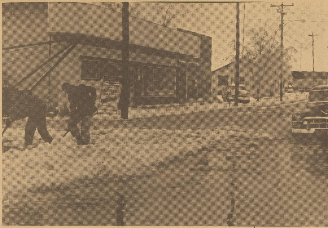
AND THEN IT MELTED -- Warming temperatures plus rain sent streets over their curbs when the melting snow, blocked by drifts kept water in the street. Above workmen try to clear a path for the water near the Jones Supply Company on Highway 60.
