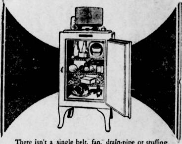
There isn't a single belt, fan, drain-pipe or stuffing box in the General Electric Refrigerator. There's nothing to get out of order. There isn't an exposed moving part. All the mechanism, built and tested in the General Electric laboratories, is hemetically sealed in a single steel casing. Come in and see these remarkable refrigerators.
