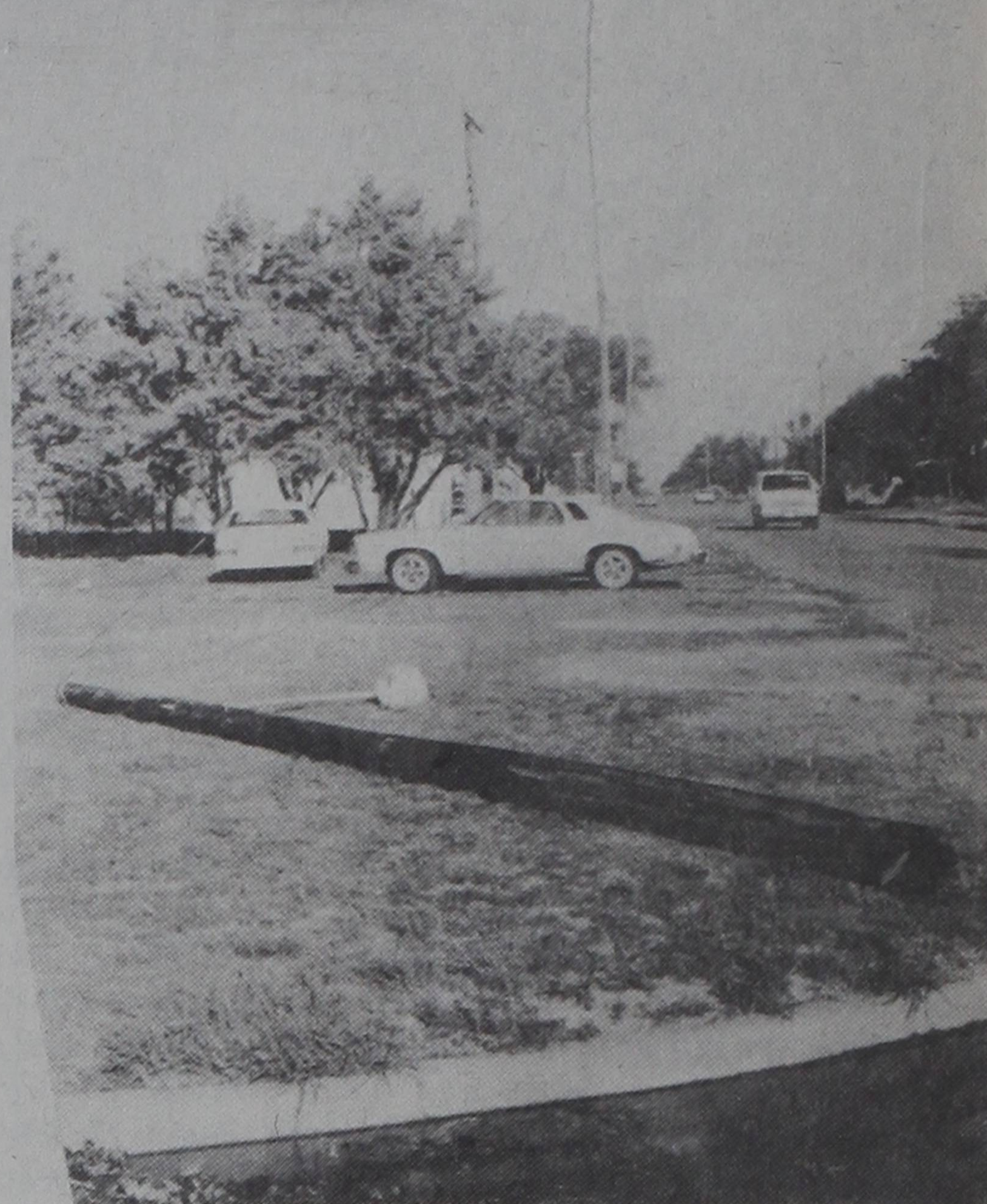
POLE CASUALTY... A power pole was a casualty of Monday night's storm, which caused considerable damage. This pole was on 14th Street on the northern edge of Friona.
