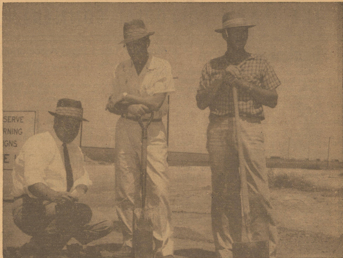
NEW STATION, RESTAURANT—Dr. Loyd Shackelford and Nelson Welch look over plans while Raymond Fleming takes in the plot of ground upon which will soon rest a Humble service station and new restaurant building. Dr. Shackelford and Welch are partners in the business venture. Fleming is the contractor.
