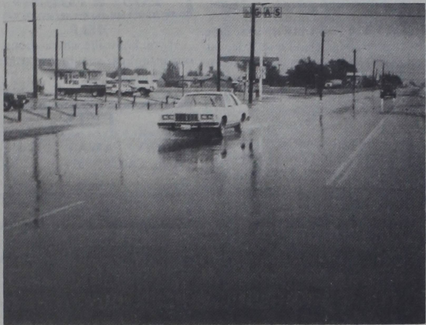
AFTER DOWNPOUR.... The outside lanes were under water Sunday afternoon on U.S. Highway 60 through Friona. At one point, the entire highway was virtually covered in water east of Main Street, with the exception of the middle turning lane.
