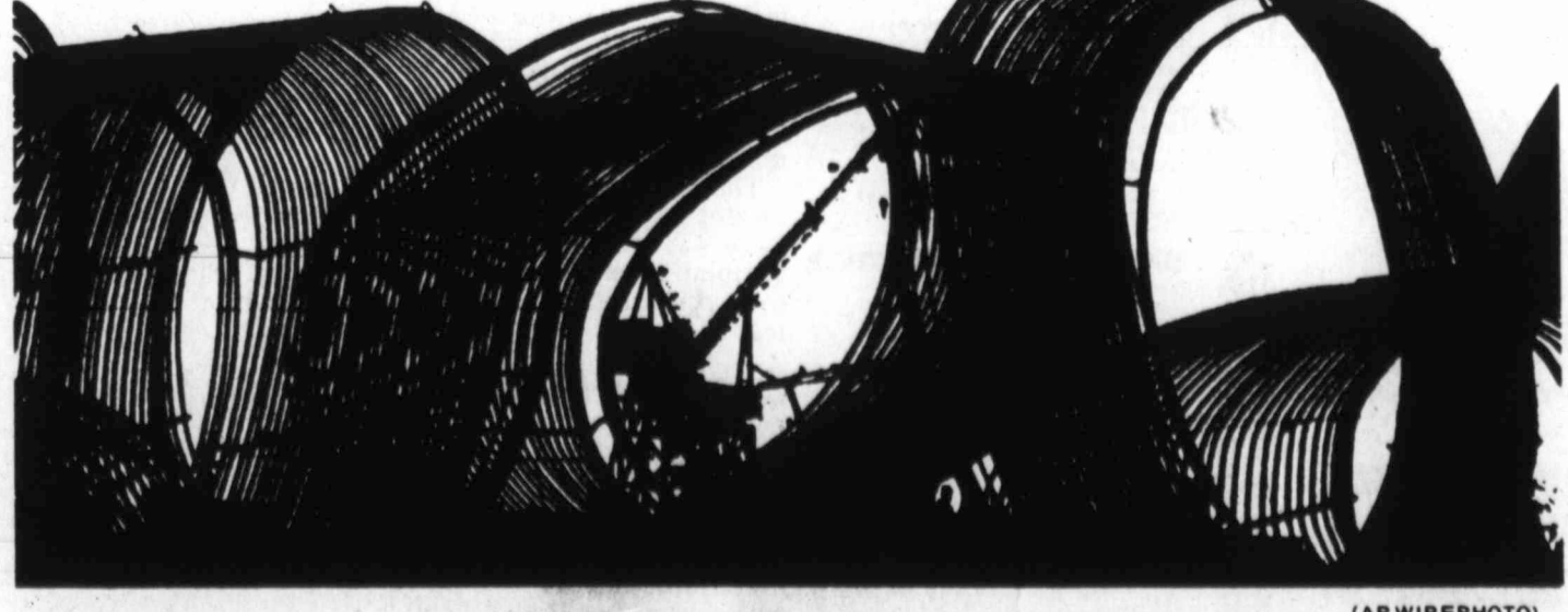
GIANT SCULPTURE? — Huge cylindrical objects are silhouetted on the skyline of the Parker Point section of Tampa, Fla. What appears to be giant sculpture is really rows of reinforced steel used in construction of concrete culverts. Background are the tall cranes of a shipyard.
