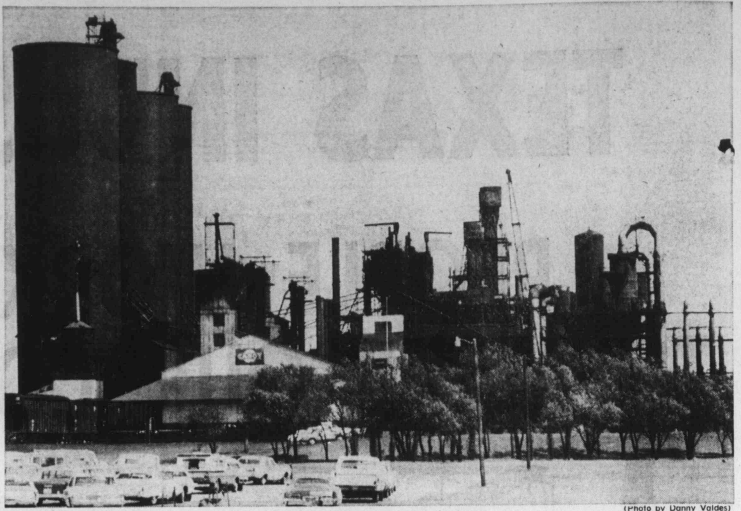
FAMILIAR LANDMARK — Cabot Carbon Company, located immediately east of Cosden Oil & Chemical Company's refinery east of town, has become a familiar landmark to West Texans. It produces carbon black, which is marketed all over the world. (Photo by Danny Valdes)
