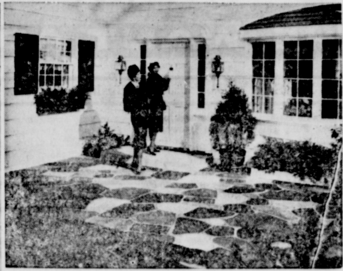
Wood windows, shutters, entranceways, and doors add charm and practicality to popular Colonial architecture. Women are turning increasingly to individually styled traditional architecture to avoid look-alike pseudo modern houses.
