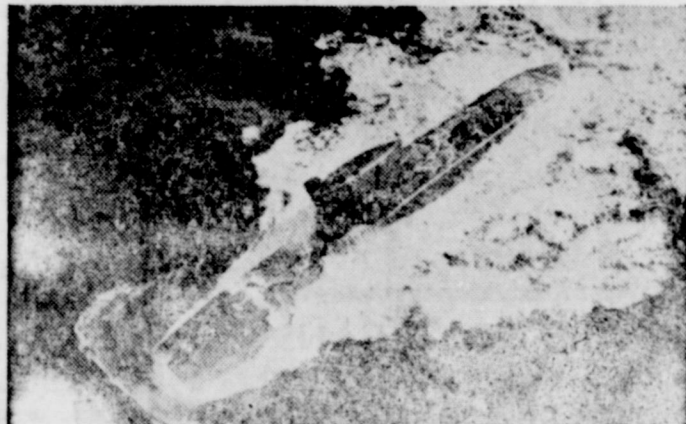
THE UNITED STATES NAVY accepted its first submarine, the USS Holland, in April of 1900, marking the beginning of the U.S. submarine service. The 54-foot long, 75-ton Holland is shown above during trial runs in Peconic Bay, L.I. Below is the Navy's newest submarine, the nuclear powered USS George Washington. Designed to fire the Polaris intermediate range ballistic missile from submerged positions, it displaces 5,400 tons and is 350 feet long. Both submarines were built by General Dynamics Corporation's Electric Boat Division, Groton, Conn.
