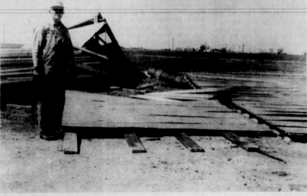
WIND DAMAGE . . . The photographs above show two instances of damage done by apparent tornado winds last Sunday afternoon near Hub. On the left is Edward (Ted) Engram, shown with the wreckage of the 18x40 storage shed which was completely dismantled. The shed is just west of Engram's home, although other buildings and objects were not harmed - even lighter objects.
