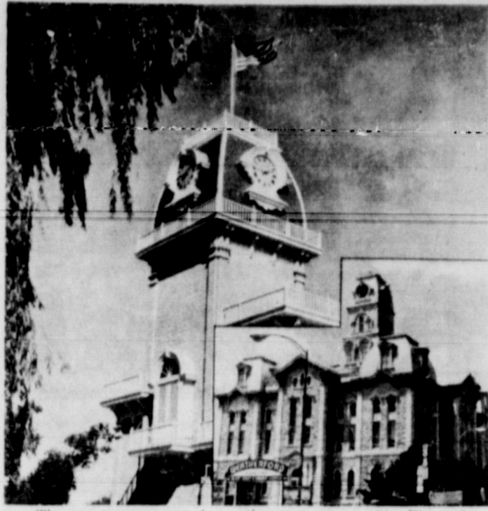
The newly constructed courthouse tower at Six Flags Over Texas looks similar to the historic Parker County Courthouse (insert) built in Weatherford, Texas in 1885. The only difference being that the Six Flags courthouse in reality is an ice plant which produces 4,500,000 pounds of ice each season for the Park's usage. After Labor Day, September 6, Six Flags will be open on Saturdays and Sundays only until the season ends on November 28.
