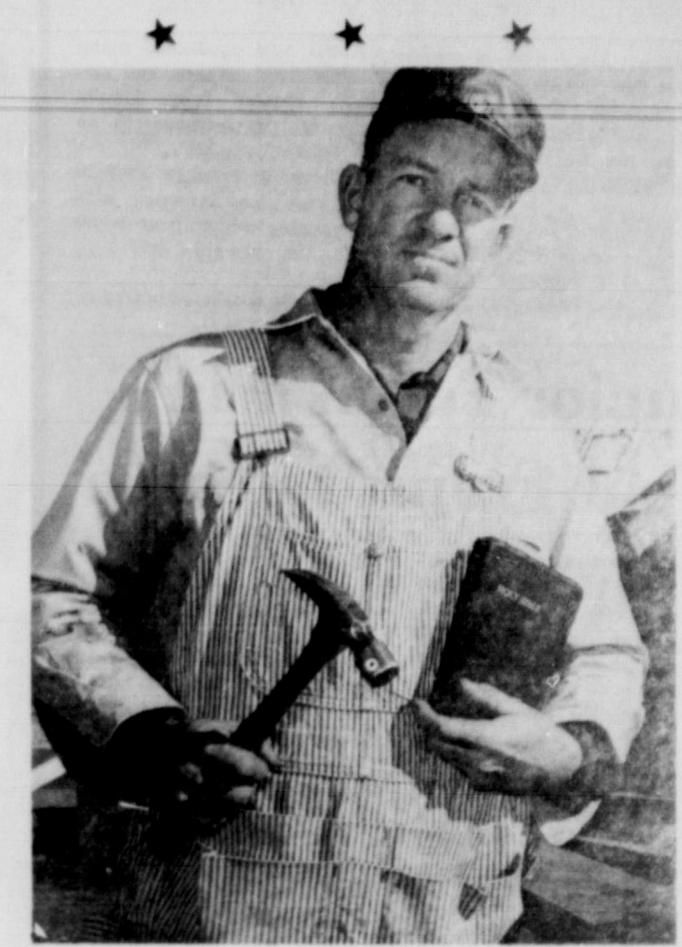
BUILDING PREACHER... Rev. Frank Baber, pastor of the United Pentecostal Church, is at home with either a Bible or hammer in his hand. He's currently serving as architect-in-charge of his church's building program.
