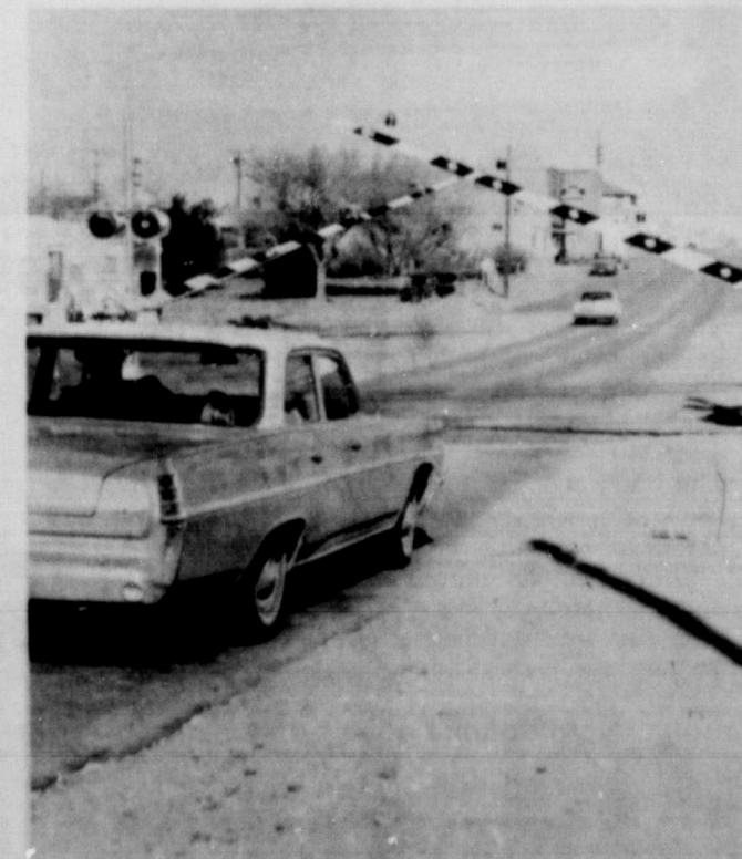
down while the train is crossing, and then raises to allow traffic to proceed across the track when the way is clear.
