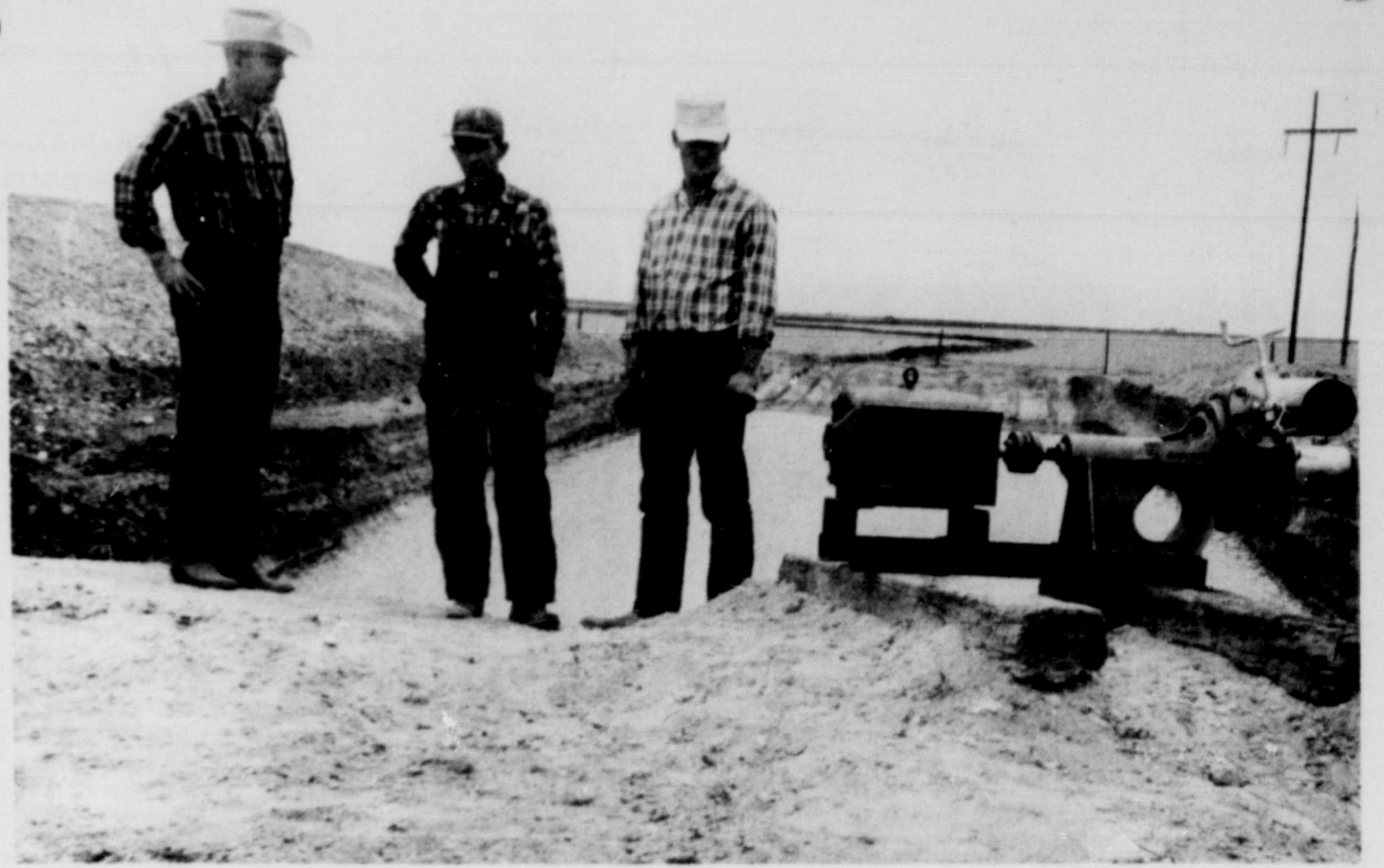
PUTTING THE FINISHING touches on a tailwater tank system near Bovina are J. D. Kirkpatrick, Buster Howard and Jim Howard. The tank is on the Jack Dunn farm, and tailwater which collects from about three farms in the vicinity will be used by Kirkpatrick in his farming operations.
