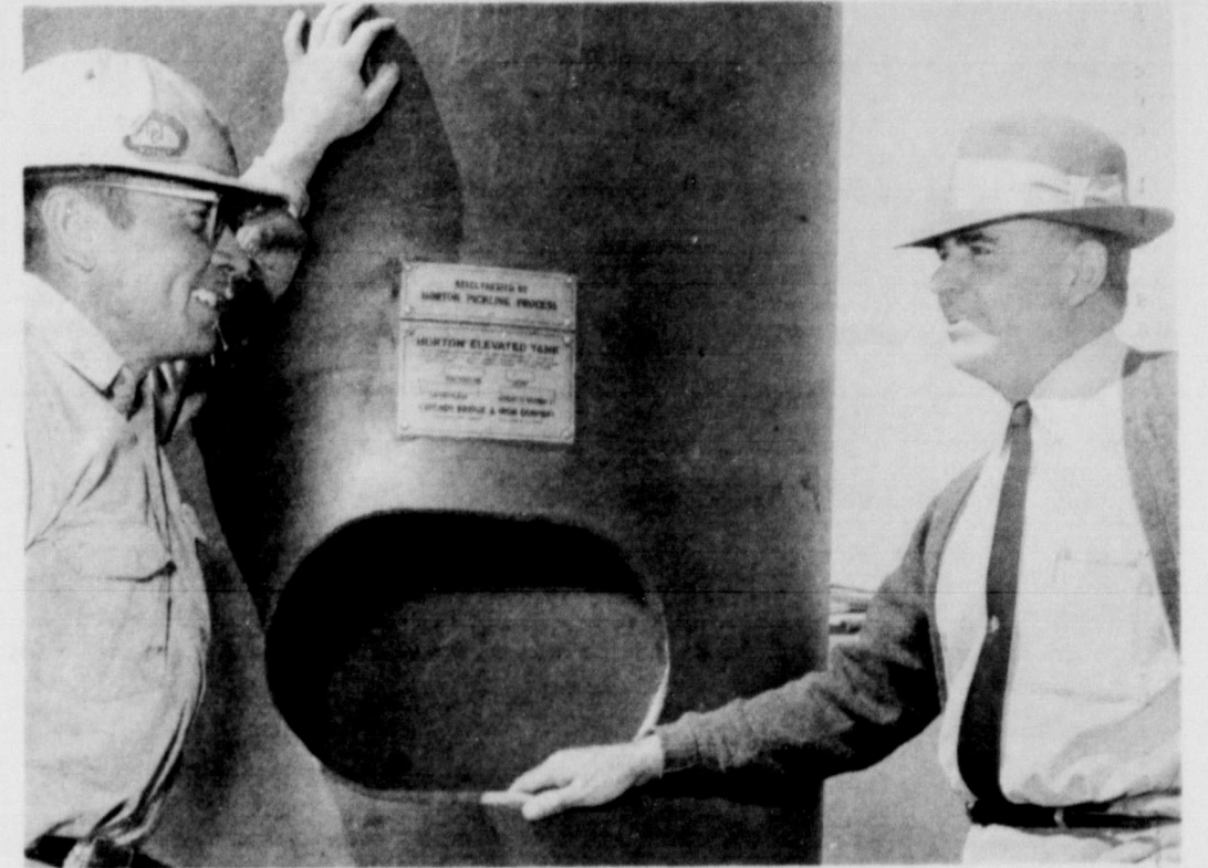
BEGINS TOWER WORK . . . Albert Bergstead, left, foreman of Chicago Bridge and Iron Company's team which will erect the new water tower in Friona, goes over his plans with City Manager Jake Outland.
