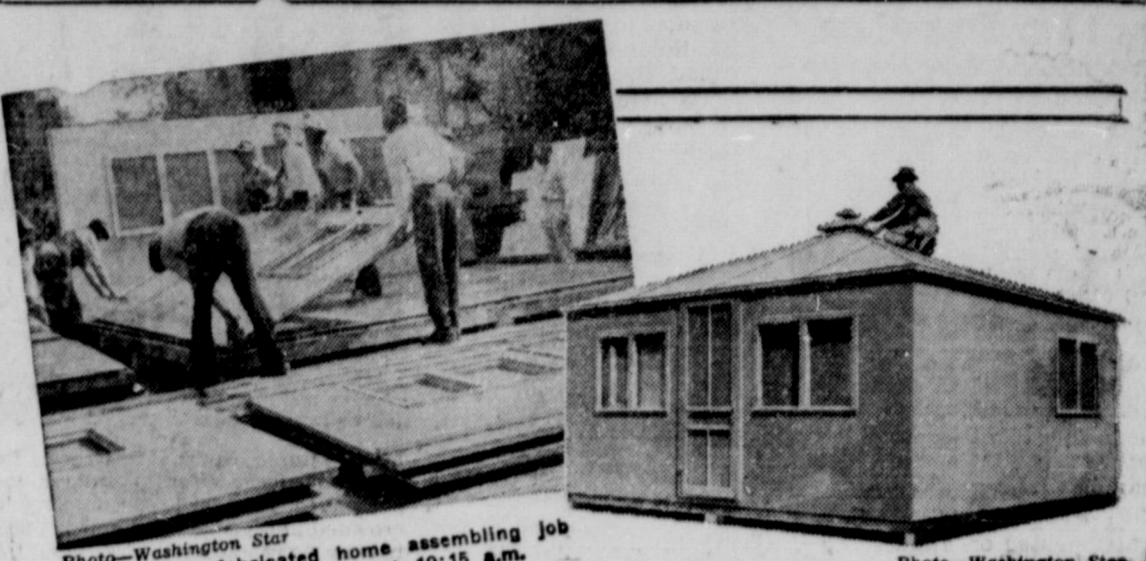
Photo—Washington Star Start of prefabricated home assembling job by inexperienced crew at 10:15 a.m.
