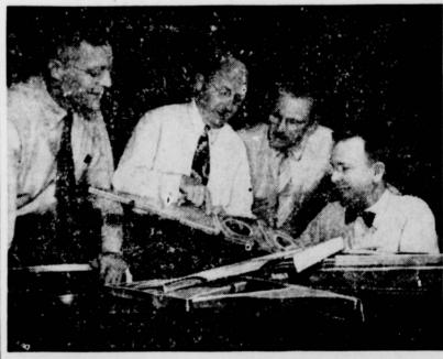
Research men of the Aluminum Company of America inspect airplane wing beams made of a newly developed aluminum alloy, "75-S." The new metal is said to have a "compressive yield strength" of 67,000 pounds per square inch, twice that of structural steel, and 50 per cent greater than the present alloyed aluminum now used in aircraft construction. The tensile strength is also very high. Experts say that "75-S" will be especially well adapted to long range bombers and fighters.
