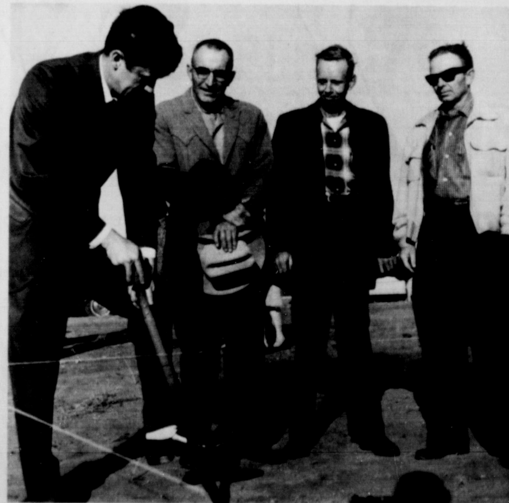
BREAKING GROUND. . . Rev. Fred Beverdorf, pastor of Friona's Redeemer Lutheran Church, turns the first shovel of dirt at ground-breaking ceremonies for the new church building Tuesday. Looking on are (left to right) Carl Schlenker, chairman of the building committee, Thomas and Frank Matlock, who are contractors for the building. (See story on an inside page.)
