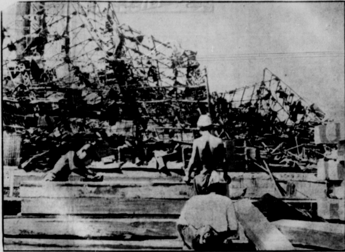
Nagasaki, second city devastated by the atomic bomb, is slowly taking shape again. Here Jap workmen prepare lumber for rebuilding homes. This area is about half a mile from the center of the blast. Twisted steel in background indicates its terrific force. (Signal Corps photo.)
