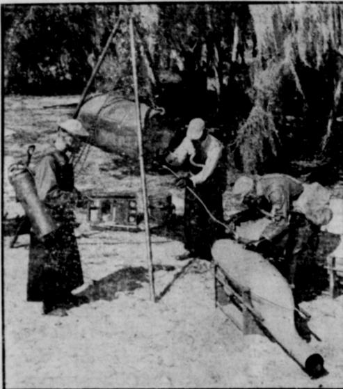
Crewmen wearing gas masks and rubber boots and aprons fill smoke tanks to be fastened to planes for a smokescreen demonstration at AAF Tactical Training Center, Orlando, Fla. Medic at left stands ready to spray water in case of mishap, for liquid smoke is corrosive. (Air Force photo.)
