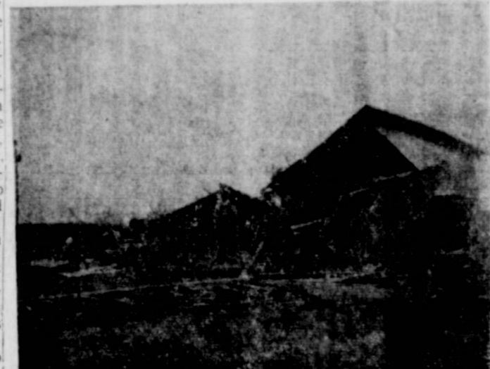
THE ORLAND HOWARD BARN , below, was treated much the same way as the Powell home though it was torn away in bigger pieces. These photographs were taken by Melvin Henry, manager of Lighthouse Electric Cooperative Inc., and loaned to The Hesperian. Lighthouse Electric crews were kept busy for a time restoring service and checking for exposed "hot" wires. Repair crews were back in Floydada by 9:00 p.m. following the storm.
