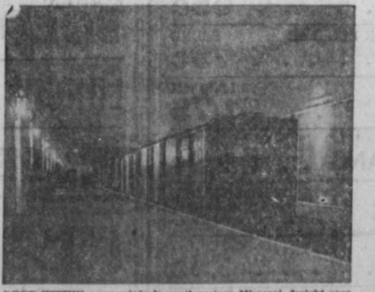
DEEP WITHIN a mountain in southwestern Missouri, freight cars await unloading of civil defense equipment to be stockpiled there for use in case of enemy attack. The siding, extending 600 feet into the mountain, can accommodate 16 railroad cars simultaneously. The Office of Defense and Civilian Mobilization facility, part of a limestone mine, contains a vast array of medical supplies and "hardware" to be used in recovery operations in the event of an attack on the United States. (Courtesy Southwestern Limestone Co.)
