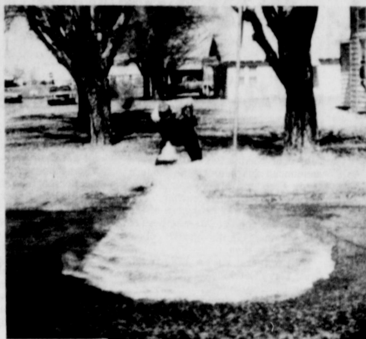
"flushing" the water mains, to get rid of sand and sediment. In addition to flushing the mains, city employees also emptied storage tanks of some 51 cubic yards of sand.
