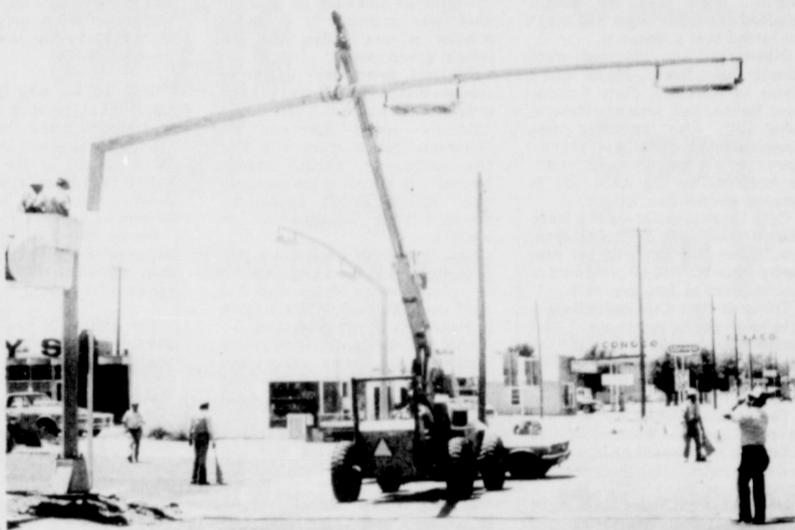
NEW TRAFFIC SIGNAL . . . The new signal lights were installed this week at the intersection of Highway 60 and Main Street in Friona, and were placed in "flashing operation" on Friday. The lights will be set in sequence operation on Monday.
