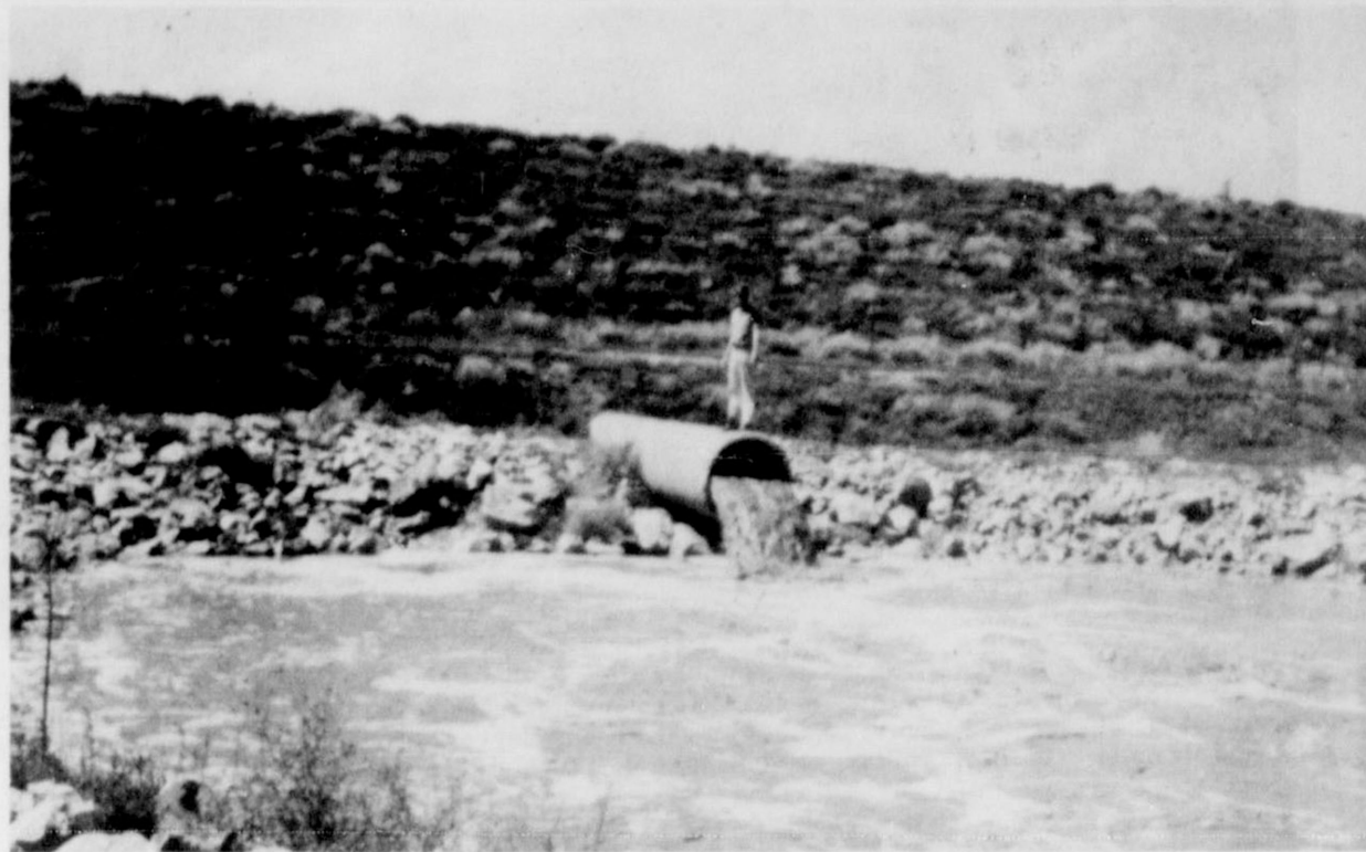
DAM FUNCTIONS.... The floodwater retention dam near Bovina functioned for the first time this week after heavy rains to the west of that area. Soil Conservation Service
