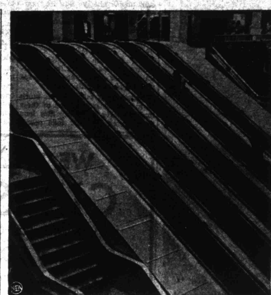
Reversible escalators run downstairs for morning rush, upstairs at night. For passengers riding 2500 buses a day, there's also the East's biggest drug store.
