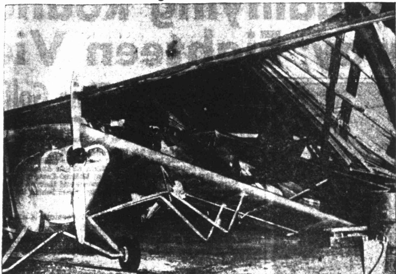
These two light planes were crushed by a collapsed hangar at Crane City Airport when a baby tornado swept West Texas, doing an estimated $150,000 to $200,000 damage. High winds, hail and heavy rains plagued several areas throughout the state.
