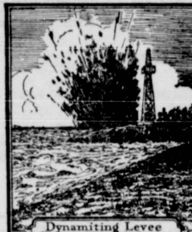
Dynamiting Levee Below New Orleans
