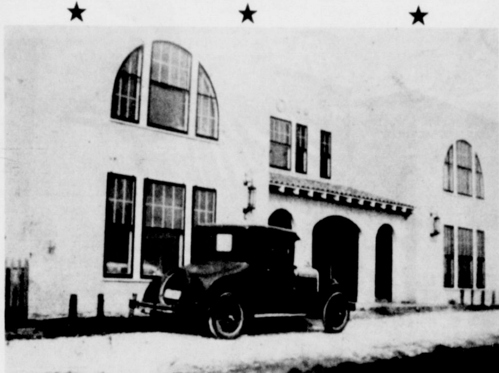
AN IMPOSING STRUCTURE....At one time, the old Syndicate Hotel, above, was perhaps the most imposing structure around in Parmer County, as it set majestically aloof east of Hub. The old hotel housed hundreds of prospective land buyers in the years gone
