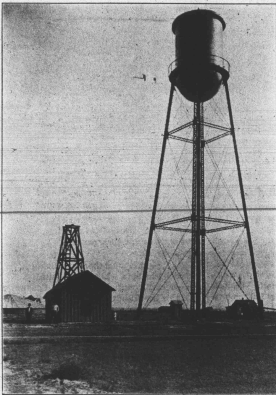
WATER TOWER AND PUMP STATION, CANYON, TEXAS
