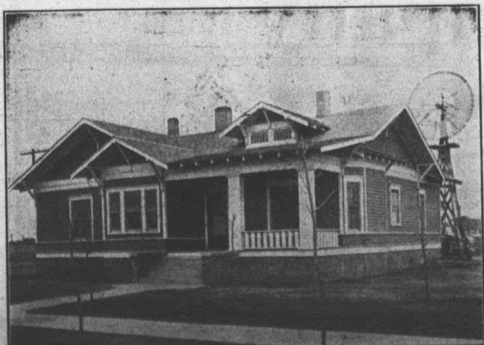
THE NEW RESIDENCE OF J. L. HUNT
