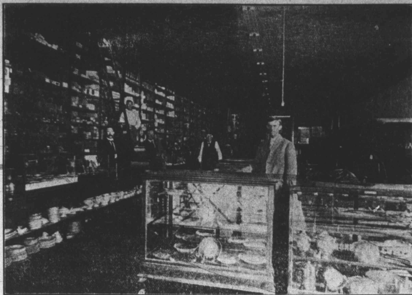
Interior View of the Thompson Hardware Company's Store
