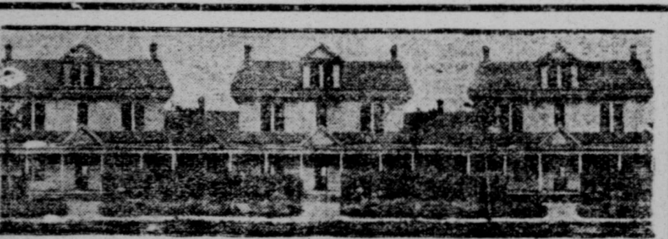
(CENTER AND WINGS COMPLETED—END ROOMS TO BE ADDED.)
