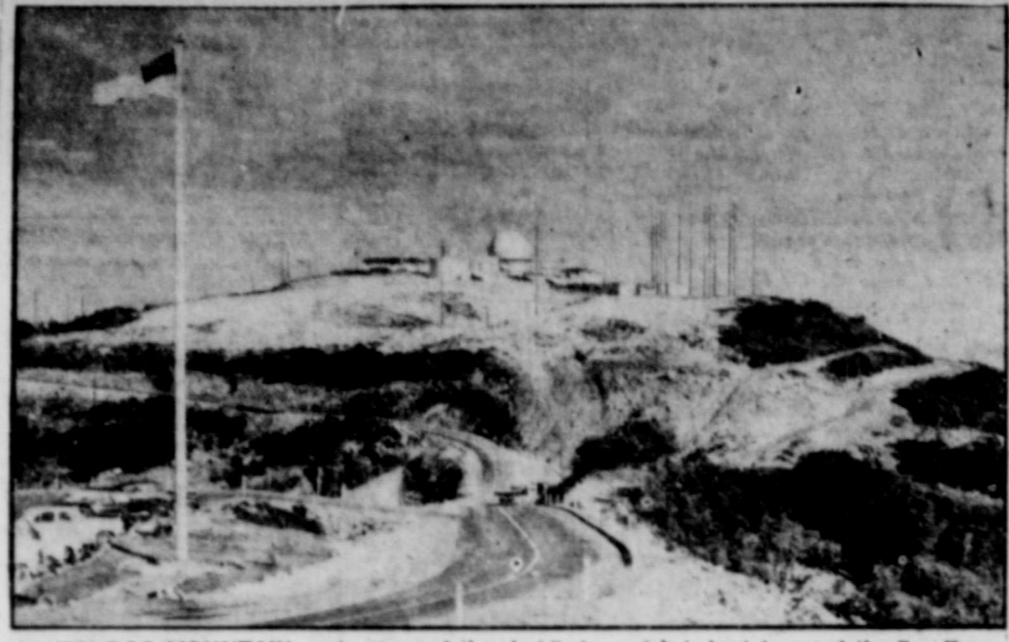
WATCHDOG MOUNTAIN — An "around-the-clock" sky watch is kept to guard the San Francisco Bay area from surprise air attack. The $3 million U. S. Air Force radar center on Mount Tamalpais picks up unidentified planes on radar screens and relays the information by radio to fighter headquarters at nearby Hamilton Field. The ball-shaped sphere at center stands 65 feet high and houses radar antennae. Wooden poles at right are 90-foot-high radio antennae towers.
