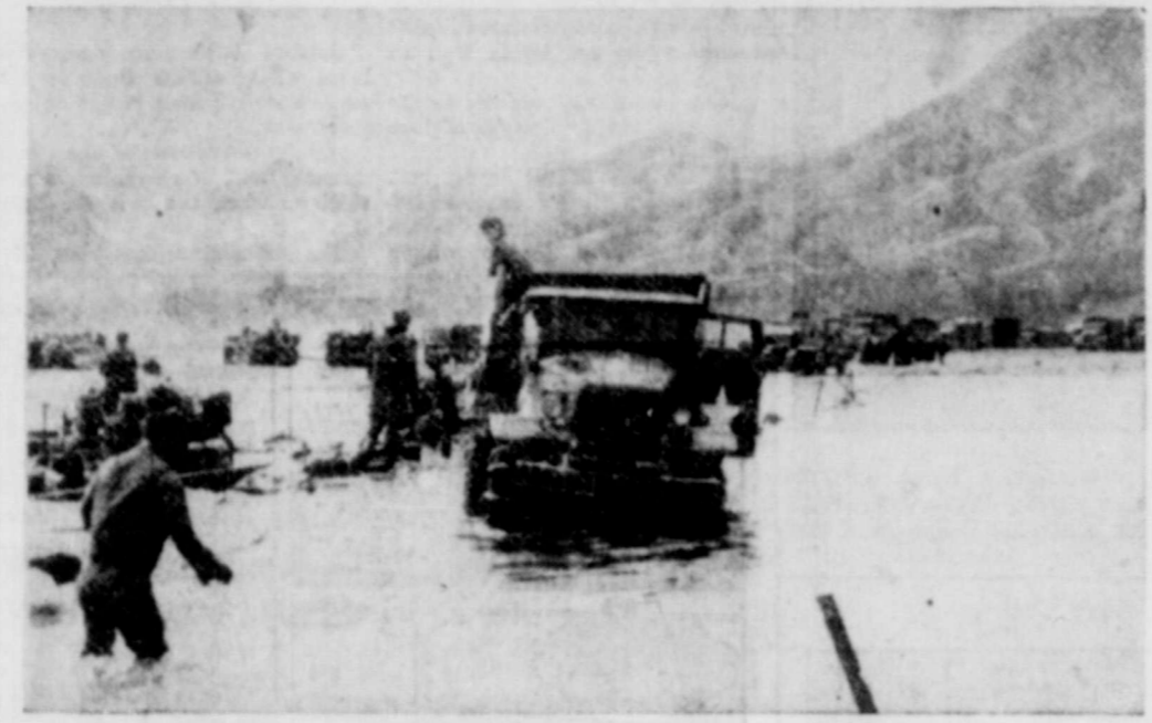
RIVER TAKES TOLL OF EQUIPMENT —The swollen Han River takes its toll of trucks and equipment as United Nations forces attempted to cross on their move north to bolster the eight United Nations Divisions which crashed forward on a 70-mile front. During a mammoth Allied offensive the Reds have lost a record 16,000 men in the first 24 hours of the drive. (NEA Telephoto).
