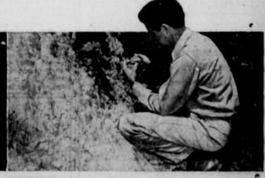
OIL GEOLOGISTS examine surface rocks in an effort to find evidences of underground formations which may contain all. Their work leads to additional exploration by other methods and to the drilling of exploratory wells. The geologist seeks rock outcrops usually found in canyons; his tools are the geologist's hammer,
