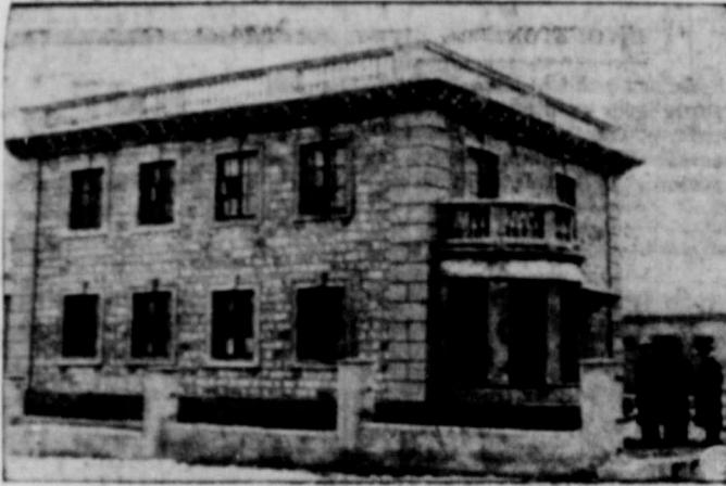
According to the Russian caption, with photo above, it shows a two-story home, constructed of blocks made from blast furnace slag. Prefabricated parts, manufactured at a special plant, were assembled within 30 days. The house is said to be the first of 200 such dwellings to be erected in Voroshilovsk.
